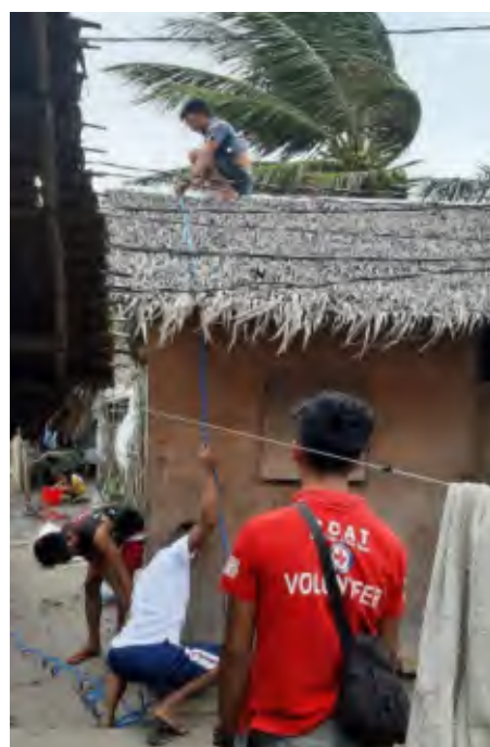
Figure 6.9 Installing SSKs in Camarines Norte (source: PRC).
